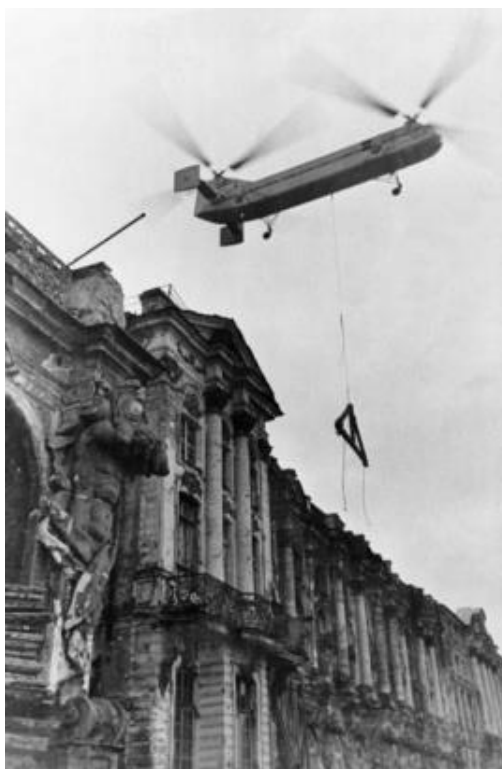
Figure 13. Installation of new trusses over the Great Hall on June 17, 1959. Helicopter commander I.S. Grigoriev
